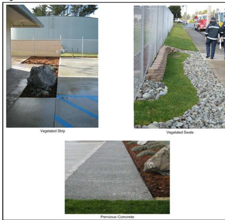
IMPs (Fire Training Facility, Eureka, CA)
