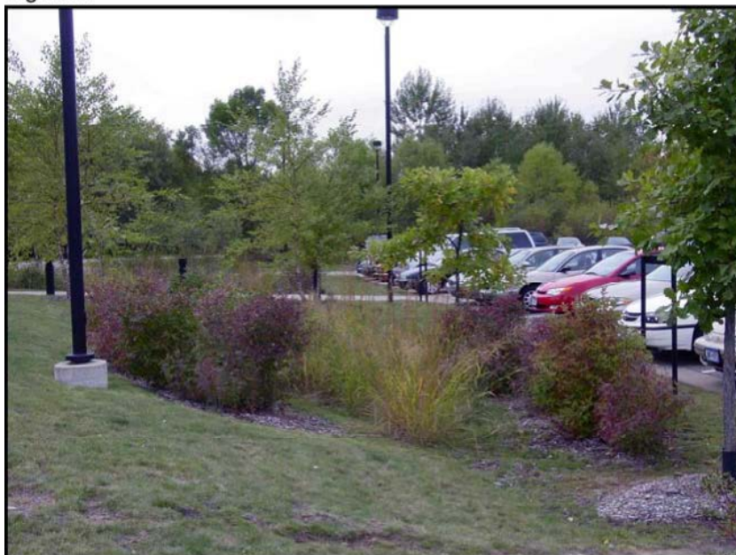
Bioretention Swale (San Diego, CA)
