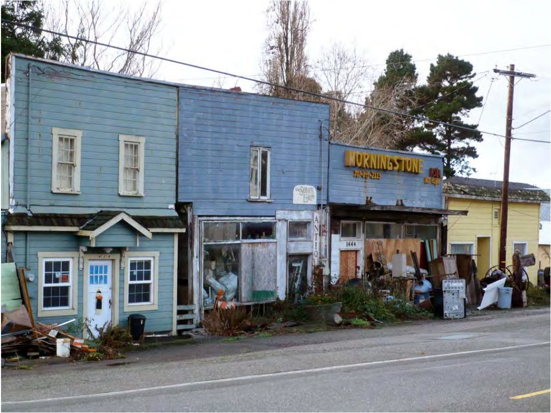
Photo of the property in a nuisance condition prior to the new sidewalk construction.
